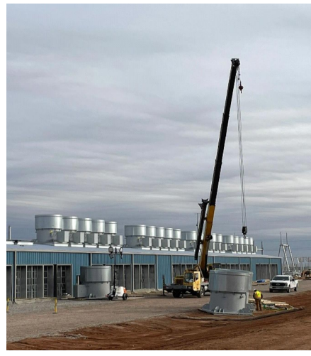
Childress – data center exhaust fan installation
