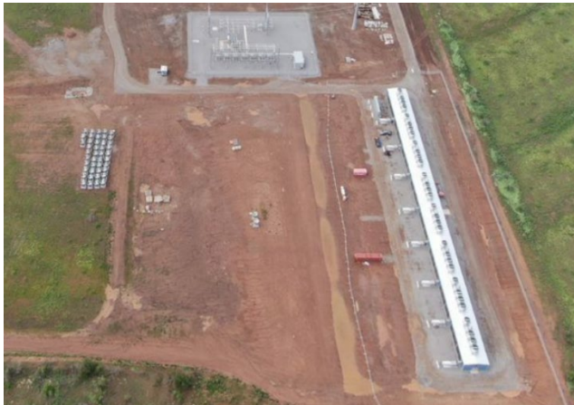
Childress (August 2023) 20MW operating data center
