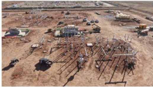
Childress – installation of transformer, structures, and electrical equipment
