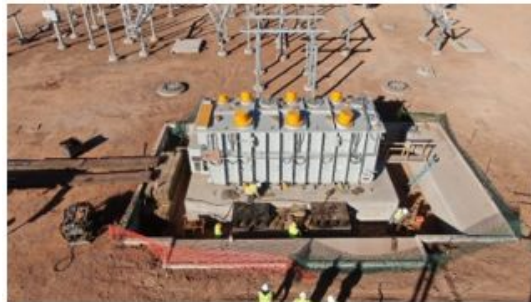
Childress – 600MW transformer set on concrete pad
