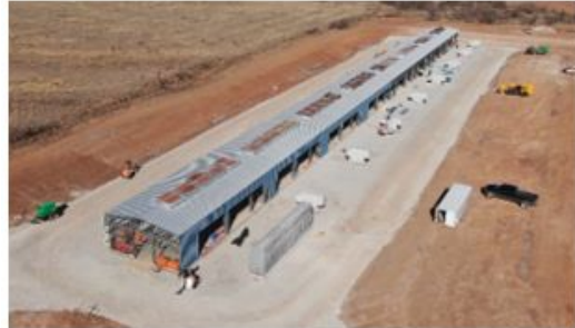
Childress – aerial view of first data center building (20MW)
