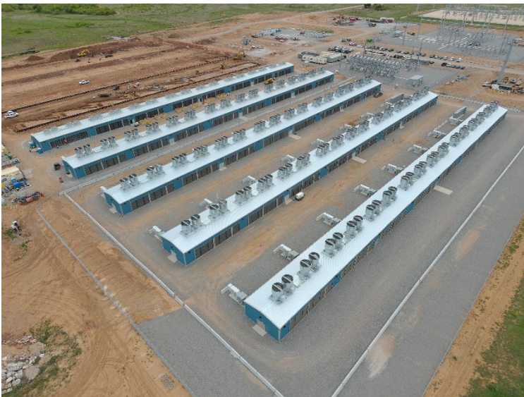
Childress construction progress (April 2024)
