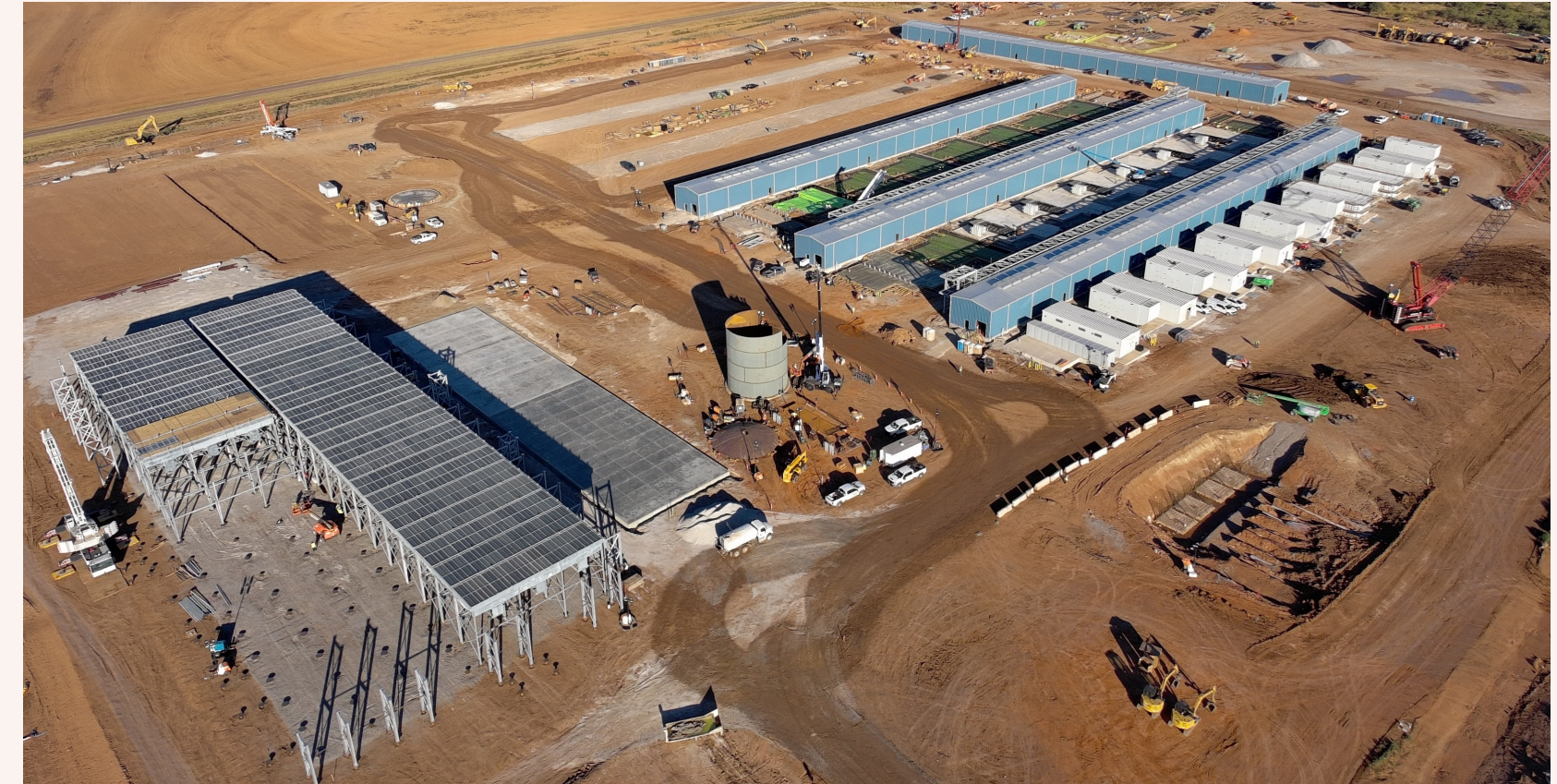
Horizon 1 construction progress (October, 2025)
