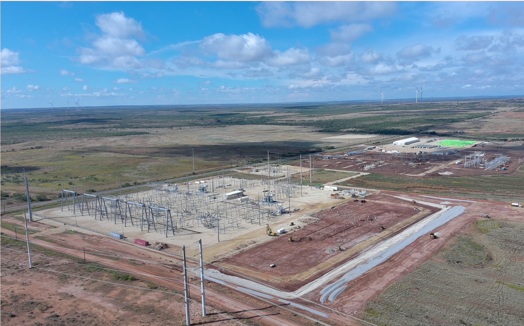
Sweetwater 1 substation construction progress (October, 2025)
