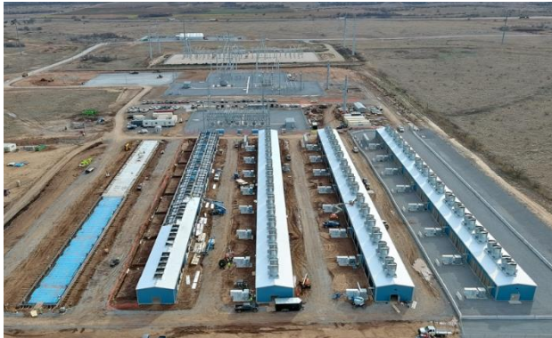
Childress – Phase 1 (100MW) construction progress
