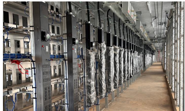
Childress – DC 2 mining operations commenced
