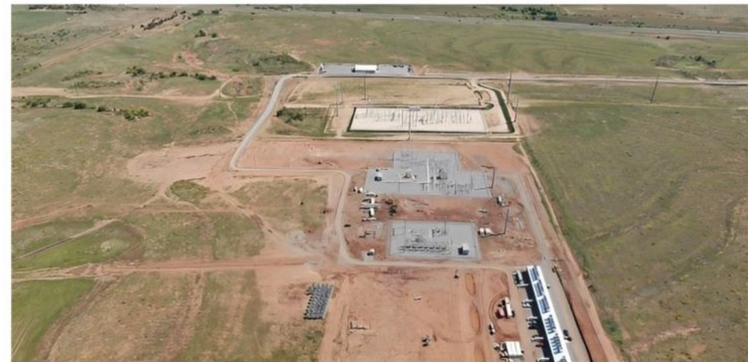
First 20MW data center operational (April 2023)
