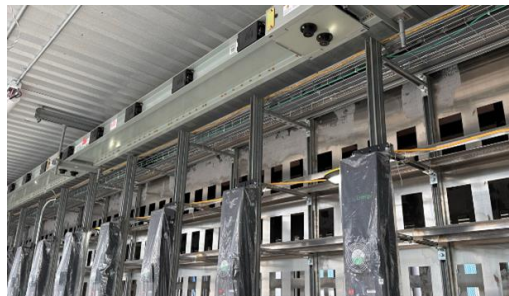
Childress – DC 2 racking & electrical installation
