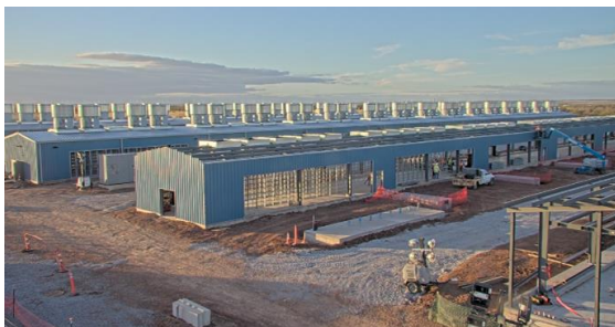
Childress – Phase 1 (100MW) construction progress
