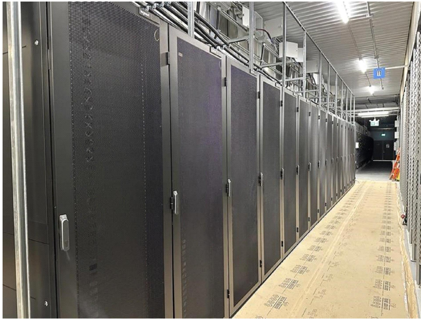
Prince George – Installation of new racks to house our fleet of NVIDIA H100 GPUs
