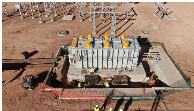
Childress – 600MW transformer set on concrete pad
