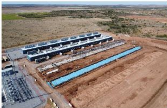
Childress – Phase 1 (100MW) construction progress
