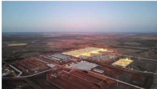
Childress Construction (Feb 2025)
