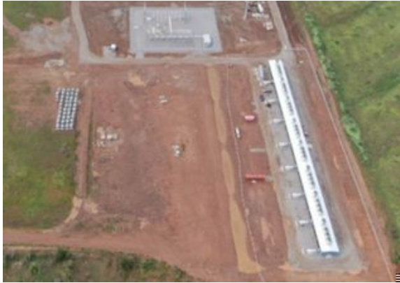
Childress (August 2023) 20MW operating data center
