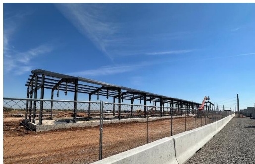
Childress – second data center primary steel structure
