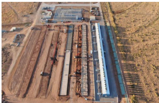
Childress – Phase 1 (100MW) construction progress
