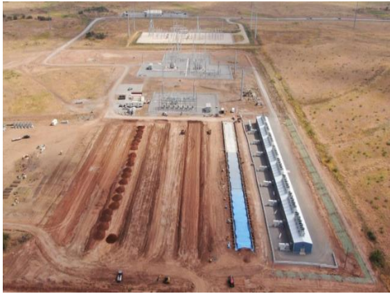
Childress – Phase 1 (100MW) construction progress
