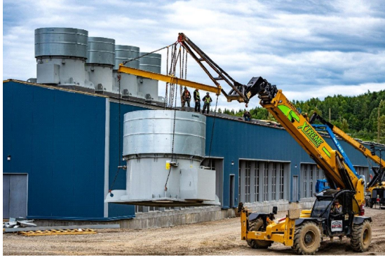
Prince George – exhaust fans being installed
