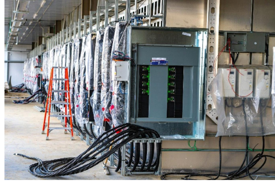
Prince George – data center internal fit out
