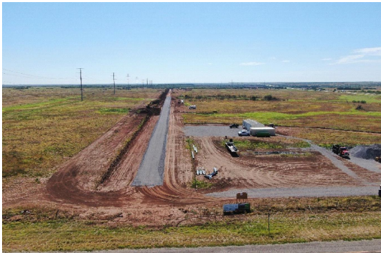
Childress – site construction office and entrance
