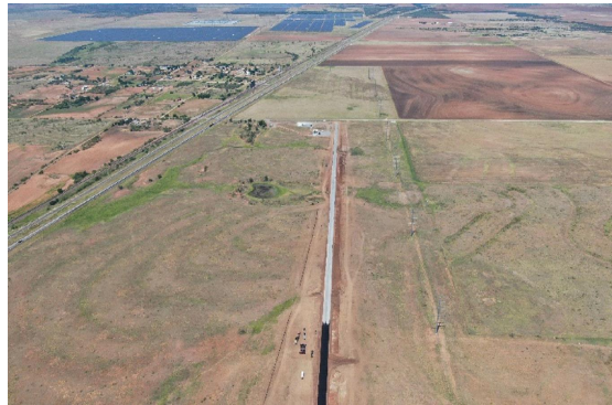
Childress – aerial view of site civil works
