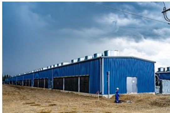
Mackenzie – second data center building
