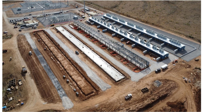
Aerial view of Childress Phase 1 (100MW) construction as of November 16, 2023
