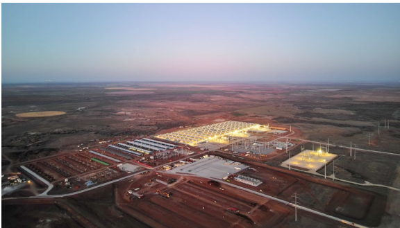
Childress Construction (Feb 2025)
