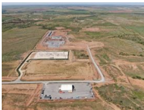
Childress – aerial view of the site
