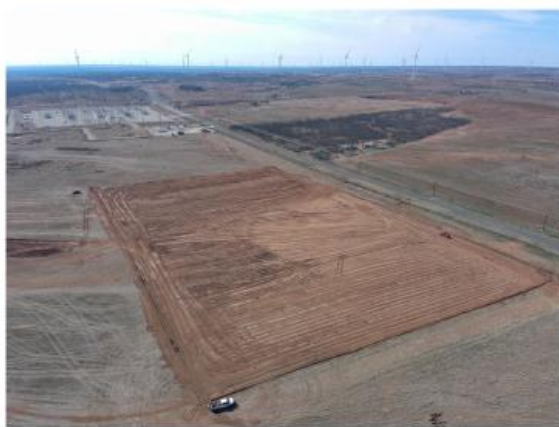
Sweetwater 1 Construction (Mar 2025)
