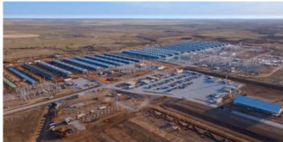
Childress Construction (Mar 2025)
