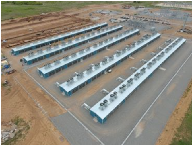
Childress construction progress (April 2024)
