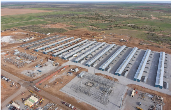
Childress Phase 4 & 5 Construction (Mar 2025)
