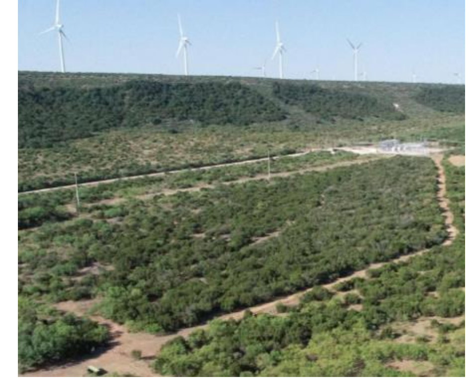
Power source: Renewables
