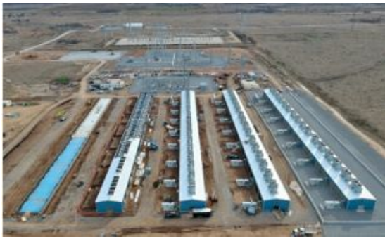
Childress – Phase 1 (100MW) construction progress
