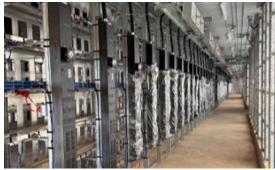
Childress – DC 2 mining operations commenced
