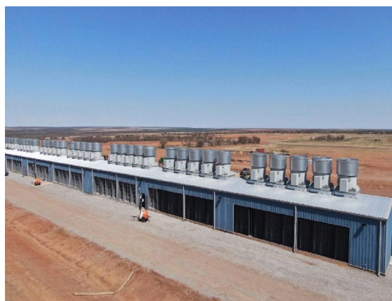
Childress – 20MW data center structural and mechanical installation complete
