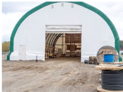
Prince George – storage facility erected
