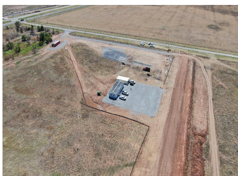
Childress – site construction office and entrance
