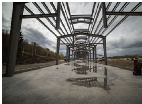
Prince George – structural steel erected for the first 20MW data center
