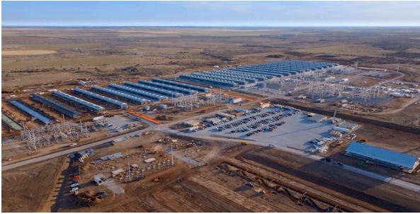
Childress Construction (Mar 2025)
