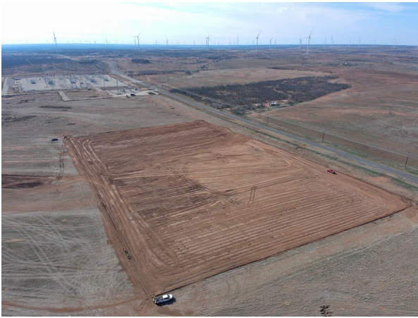
Sweetwater 1 Construction (Mar 2025)
