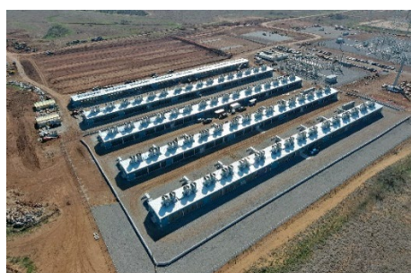
Childress Phase 1 (100 MW) construction progress
